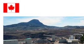
New Afton Mine ●●
