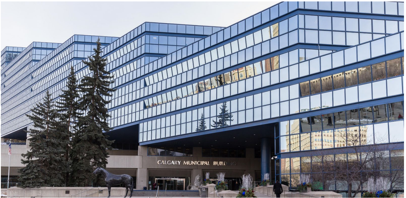
Figure: Calgary Municipal Building
